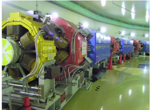
Fig. 5. All magnets have been installed in the RCS tunnel.
