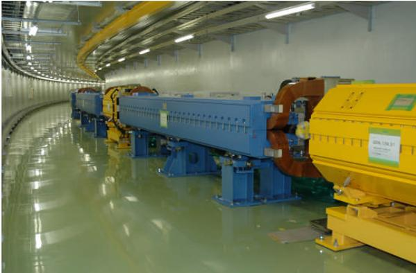
Fig. 7. All magnets have been installed in the MR tunnel.
