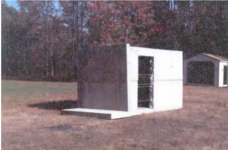
**Figure 1. Photograph of the Concrete Room Radiation Shield with Extra Side Wall.**
